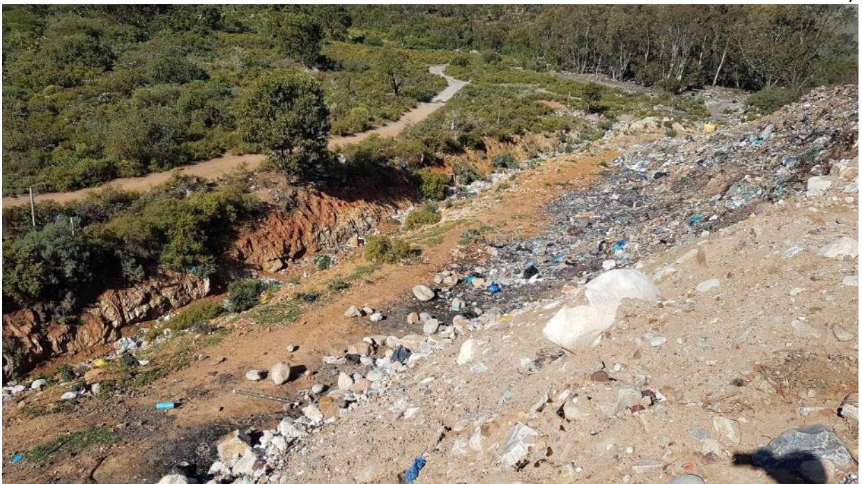
Photograph 14: Uncovered waste on slopes of the WDF in close proximity to the stormwater channels and as a result stormwater channels are filled with waste
