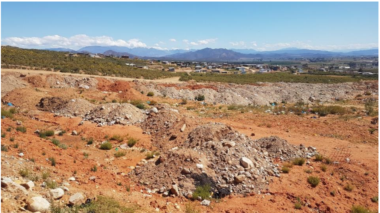
Photograph 18: Rubble stockpiled north west of the WDF to be used as cover material on the landfill site
