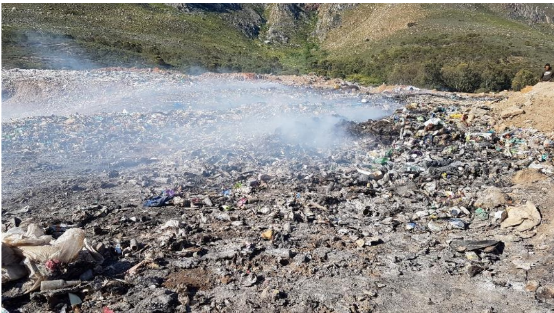
Photograph 10: Uncovered waste and burning of waste on the WDF
