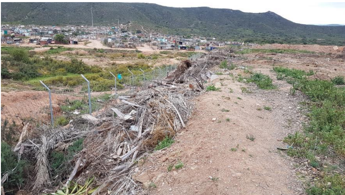
Photograph 6: Edge of the waste body with steep slopes and garden waste with thorns stockpiled against the fence to prevent community members entering the WDF. Note that the houses within the WDF buffer zone.
