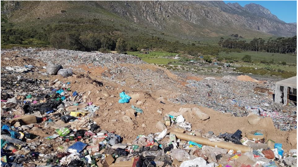
Photograph 13: View of the uncovered waste surrounding the MRF which inhibits movement of staff and vehicles around the MRF and onto the waste body
