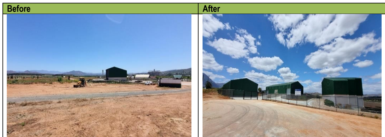
Photo: Completed Material Recovery Facility, Ashton
