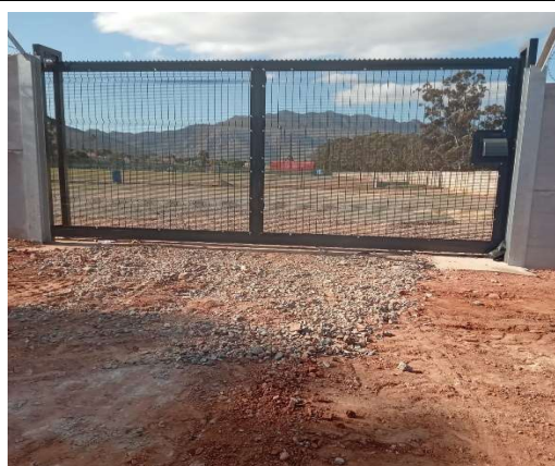
Photo: Portion of Cogmanskloof sport ground, Ashton boundary wall completed.
