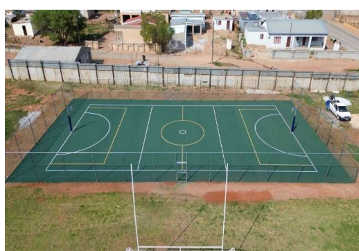
Photo: New Netball court construction Zolani, Ashton.
