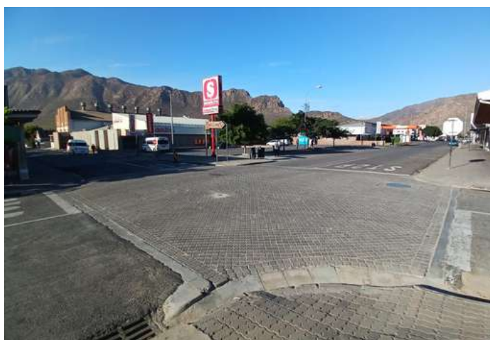
Photo: Bath and Mark Street intersection
