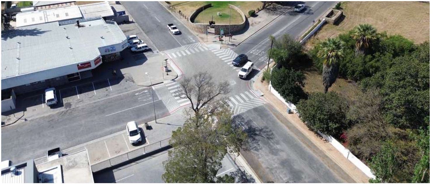
Photo: Aerial view of the upgraded Bath and Cross Street intersection in Montagu.
