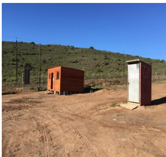
Photo 6.29: Security outhouse and ablution
