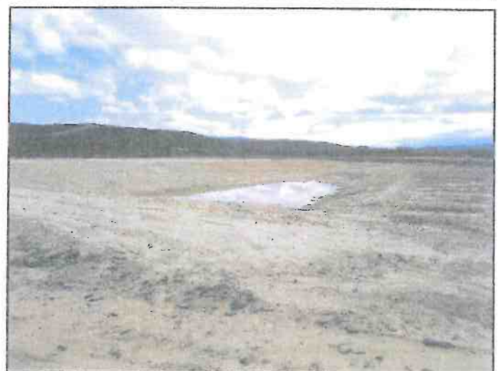
Top storm water dam
