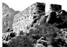
Fort Sidney – strategically positioned above the narrowest section of the Cogmans Kloof pass, guarding the road below.
