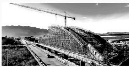
A view of the new Ashton Arch under construction, with the previous bridge still in use.
