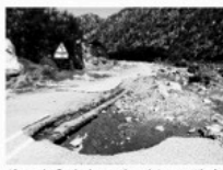
After major floods, the pass through Cogmans Kloof was impassable and emergency road repairs were undertaken each time. The new road has a higher alignment in many places which improves its resilience against flood damage.
