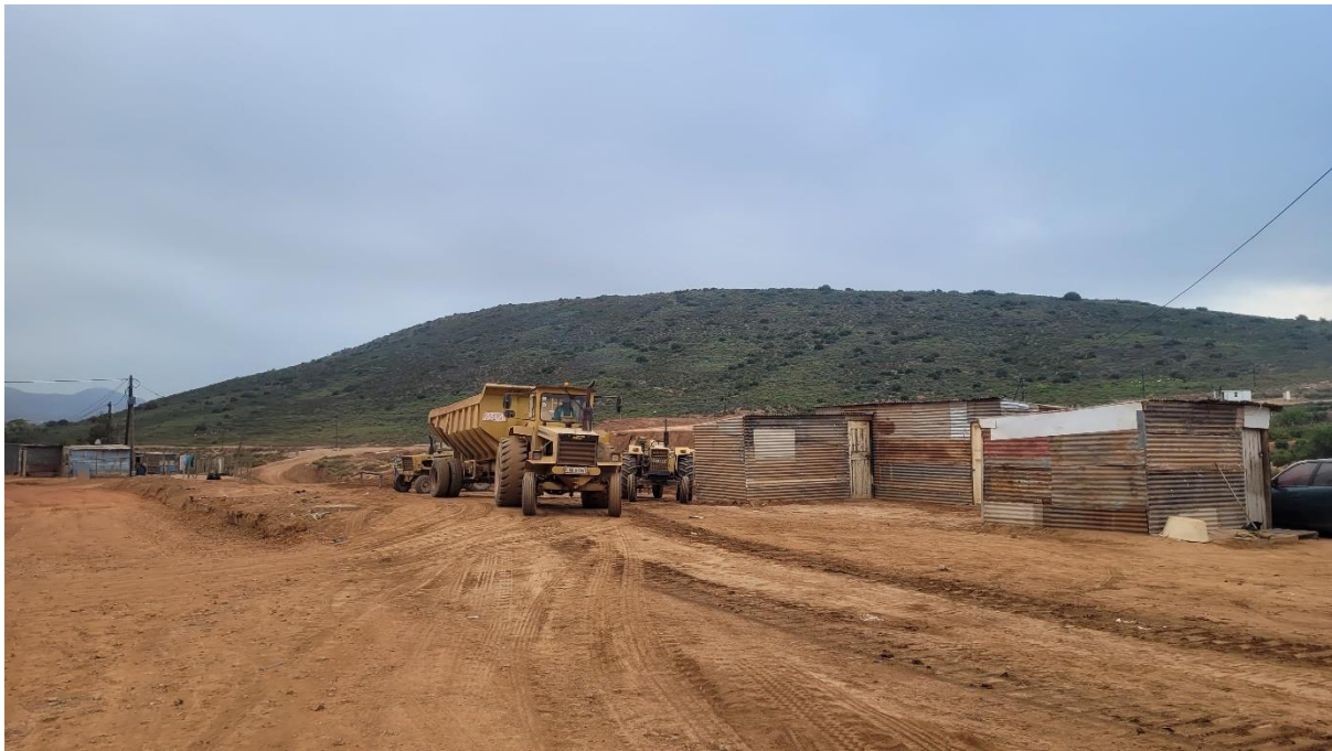
Figure 6.36: Construction vehicles in Boekenhoutskloof
