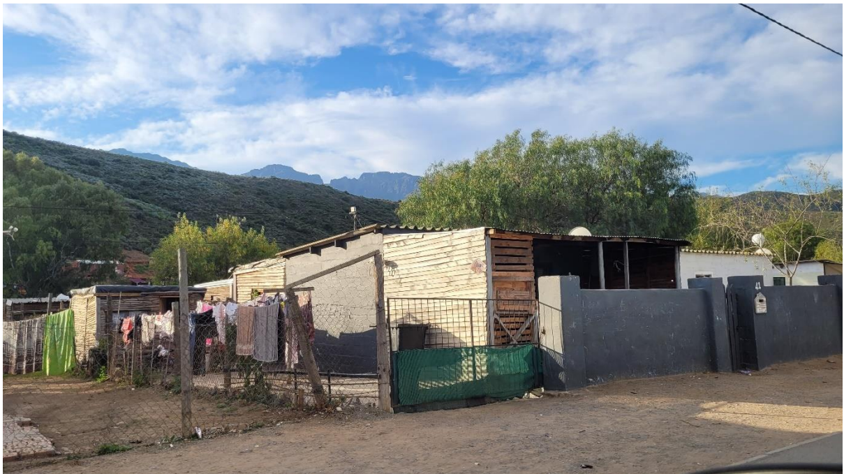
Figure 6.5: Backyard dwelling in Droëheuwel
