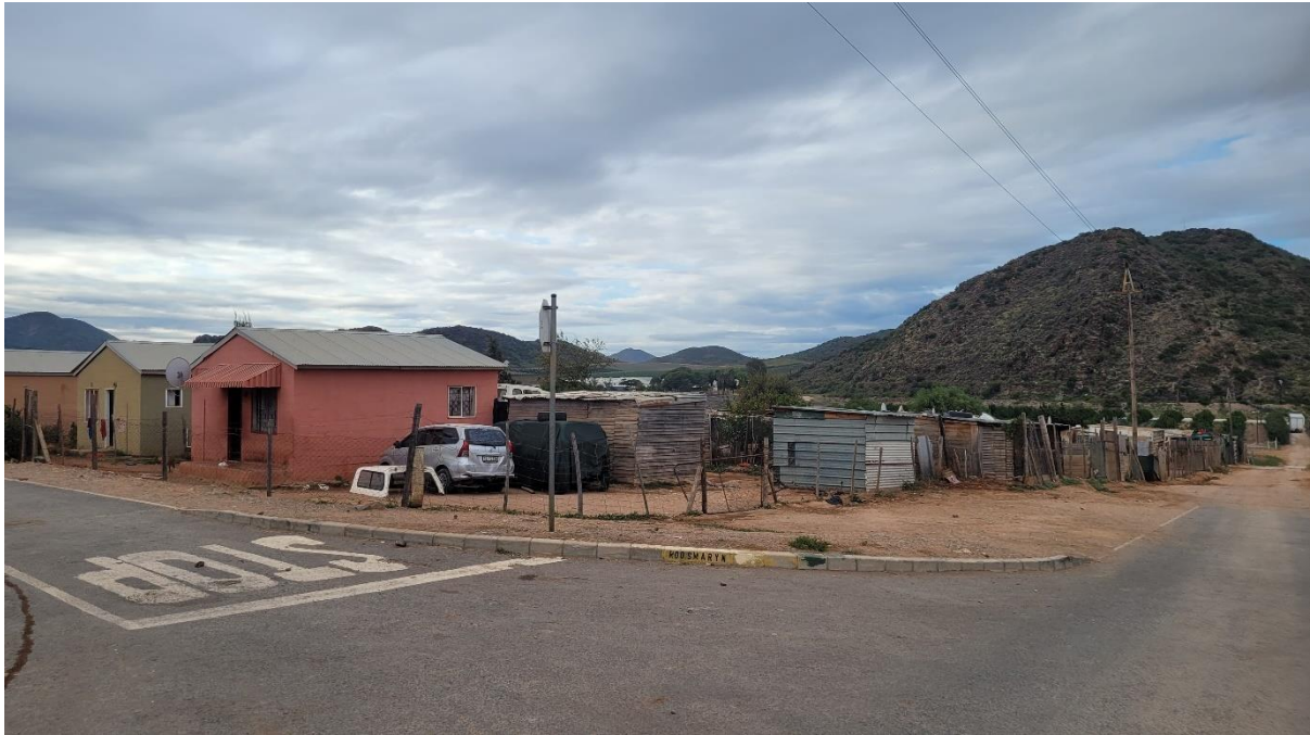
Figure 6.45: Mix of housing typologies in Mandela Square
