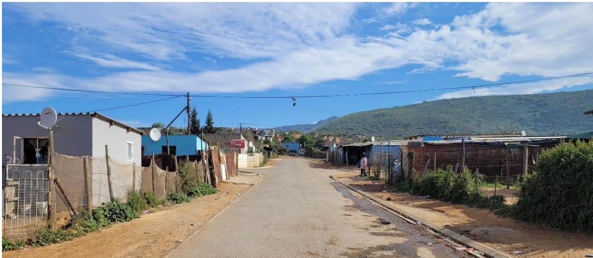
Figure 6.4: Street view in Môreson
