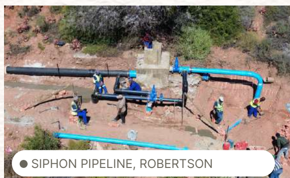
● INSTALLATION OF PUMPS AT RESERVIOR
