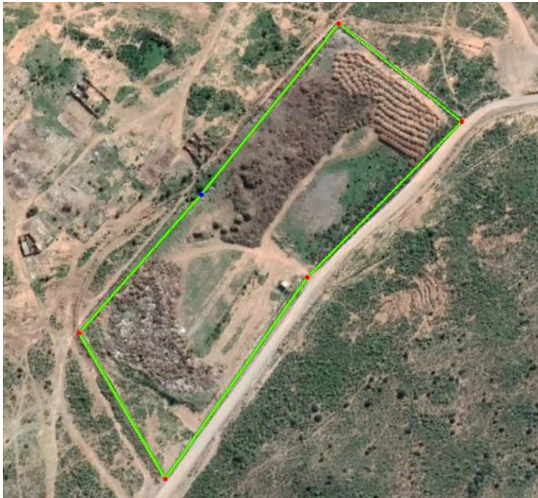
Figure 4-12: Bonnievale landfill site (Google Earth image: 2020)
