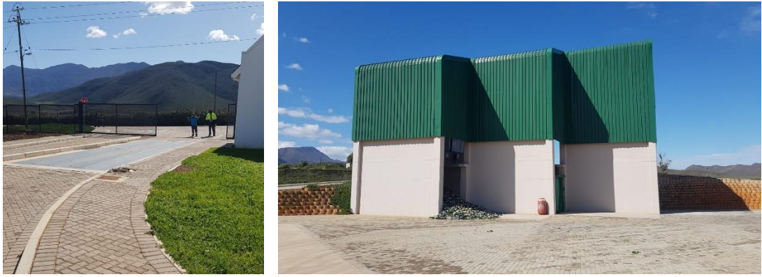
Figure 4-23: Ashton transfer station with weighbridge
