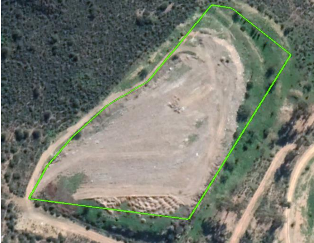
Figure 4-17: Montagu landfill site (Google Earth image: 2020)
