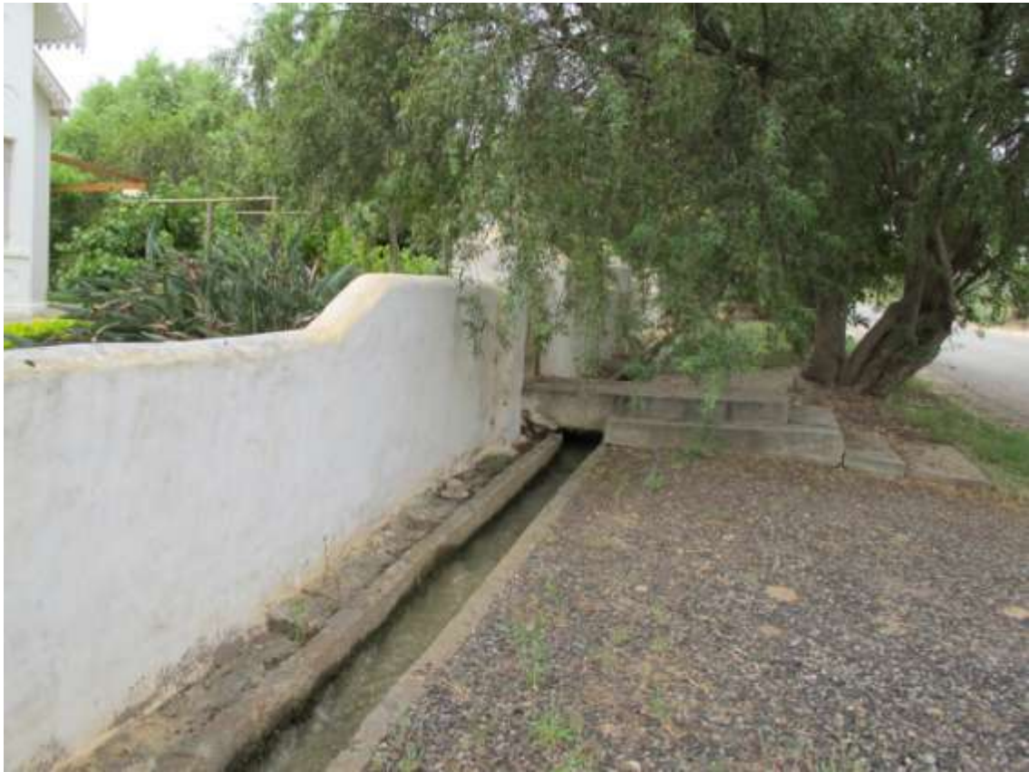
Water channel which is part of the road system on major routes
