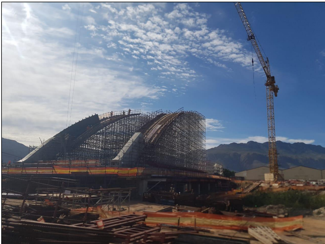
Photo of the support work to arch being erected
