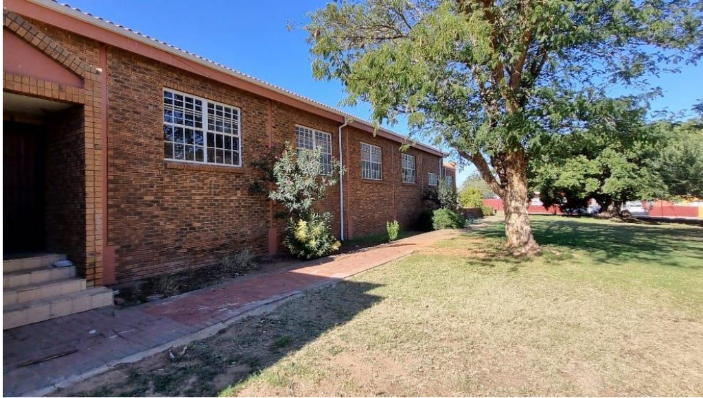
Zolani Community Hall – Replacement of Gutters & Downpipes
