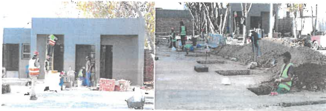
Upgrading of Robertson Informal Trading area
