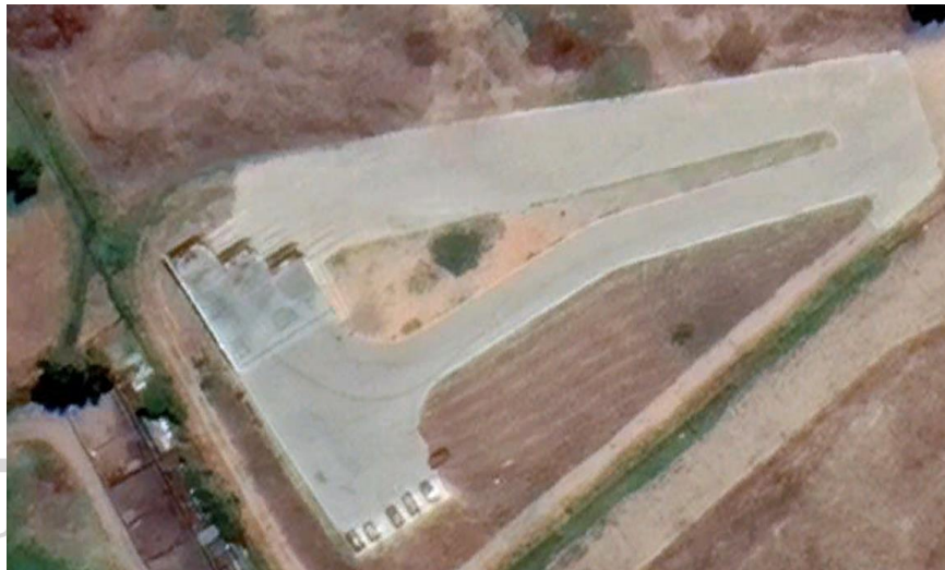
Robertson Transfer station
